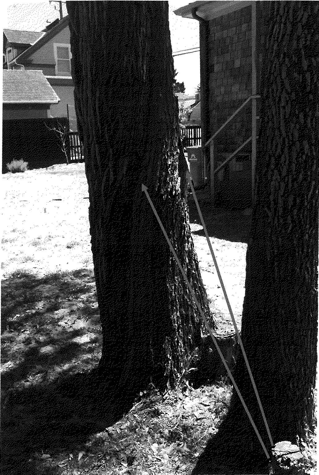
Base of tree #592 and #591; #592 has decay in the stem within the seams observed
